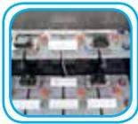
High quality battery bank. The Battery Cell Level Control system (BCLC) developed by NSE Ltd is used for the precise control and maintenance of the storage battery for many years of trouble-free service.
